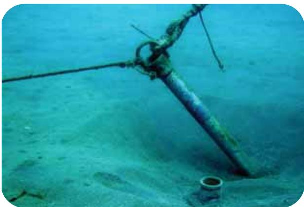
A 2-m long, heavy 5–7 cm diameter galvanized metal pipe hammered diagonally into the seabed being used as an anchor for a floating nursery above a sandy bottom (S. Shafir).
