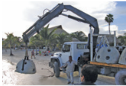
The deployment of artificial reef structures used to standardize the types of surfaces that corals may settle upon. These are being used by the RRWG in all COE locations. ©K.Kilfoyle.
